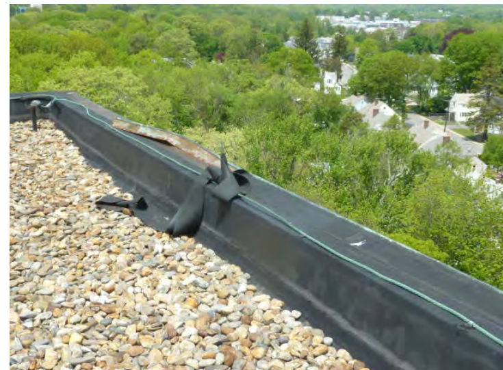
Flashing failure is cause of active leak below.
