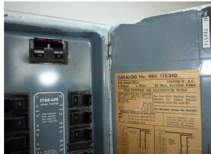
Stab-Lok electric panels and original thermostats are shown to be replaced immediately.
