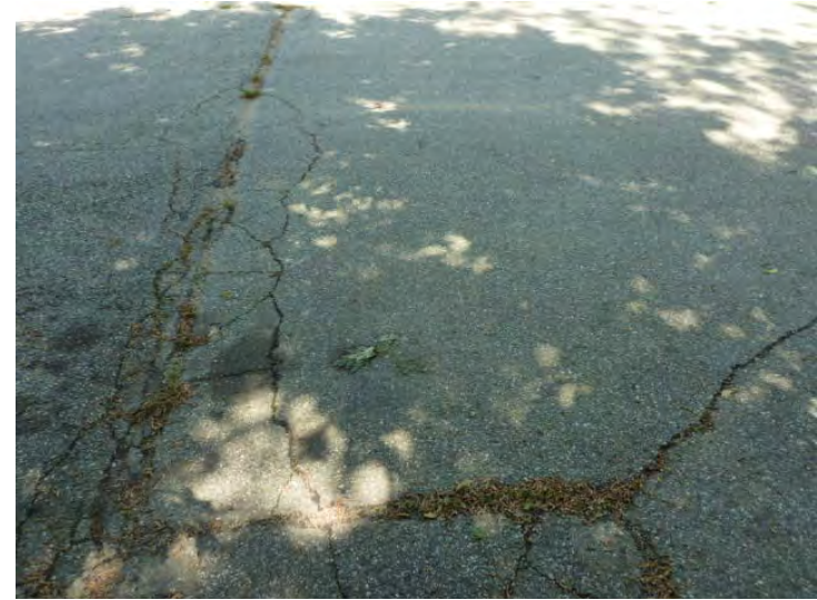
Typical cracking and sub-base failure.
