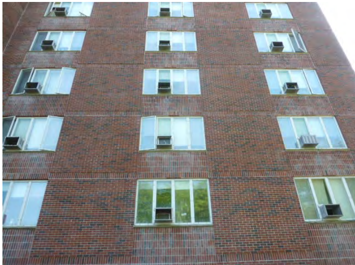
Historic efflorescence at brick panel below each concrete window sill indicates moisture penetration into the wall at the sills.
