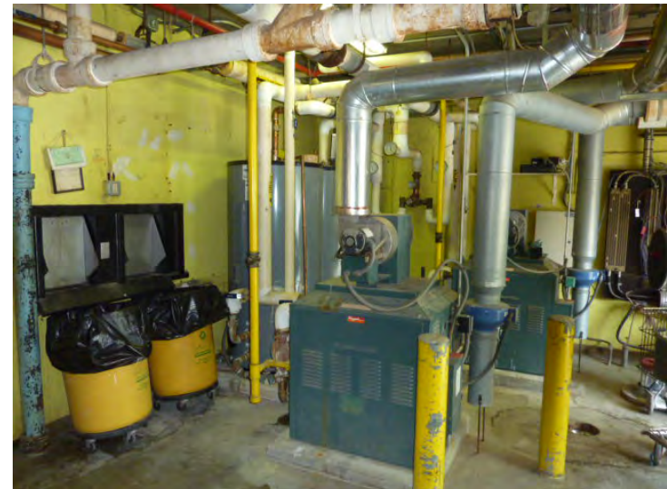
Domestic hot water boilers serving the entire building are failing and shown to be replaced in Year 1.
