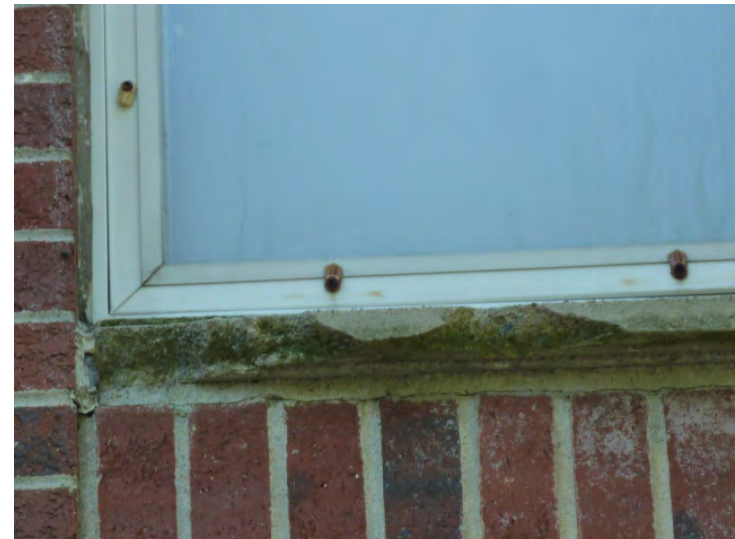
Deteriorated concrete sills at windows are shown to be repaired early in the plan.
