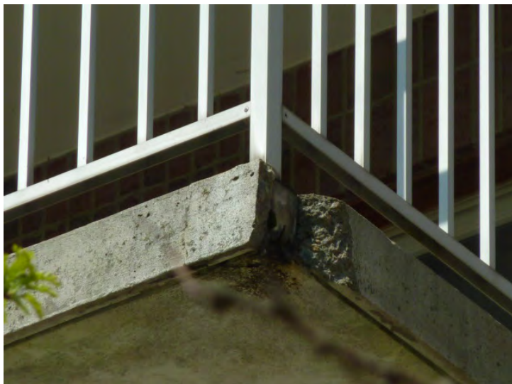
Typical failure at concrete corner at balconies is shown to be repaired.
