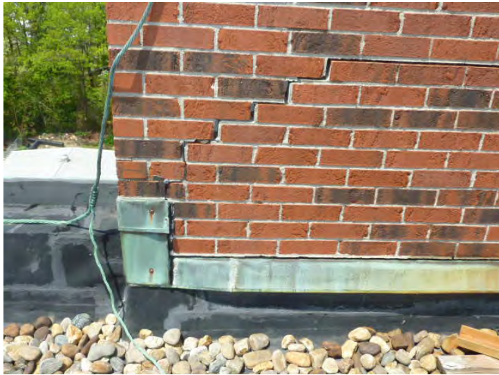
Typical step cracking and other brick failures at several select locations are shown to be repaired.
