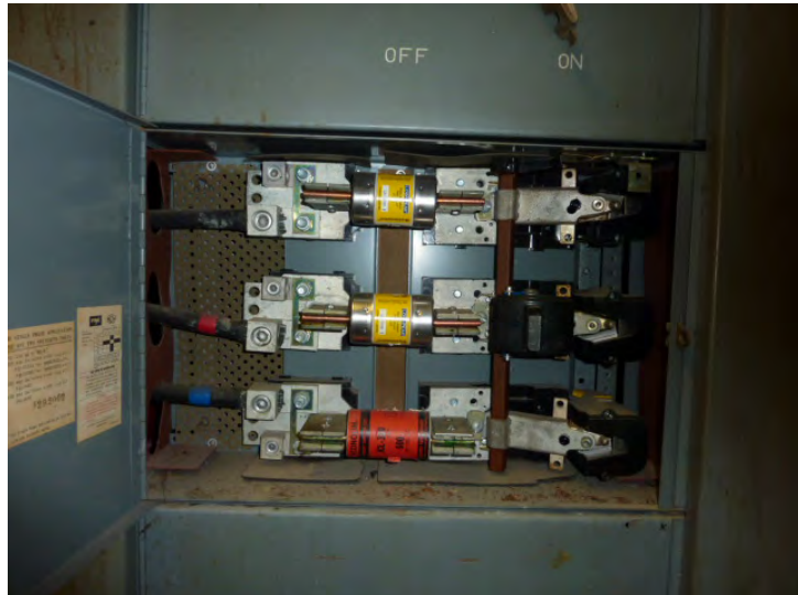
Original fuse panels are obsolete and scheduled for replacement.
