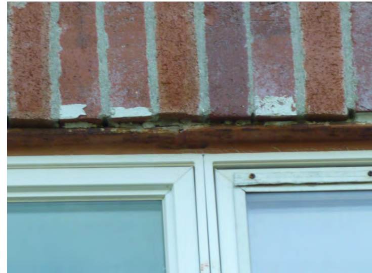
It appears sections of caulk were subsequently removed at entire stacks of windows to allow for the wall to drain as designed.
