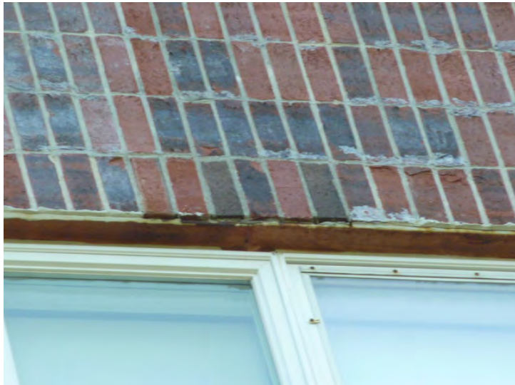
Severe efflorescence at window head where weeps appear to have been caulked closed.
